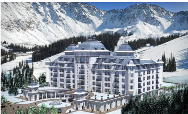
Construction fee – circa £50million Client: Pasha Construction
