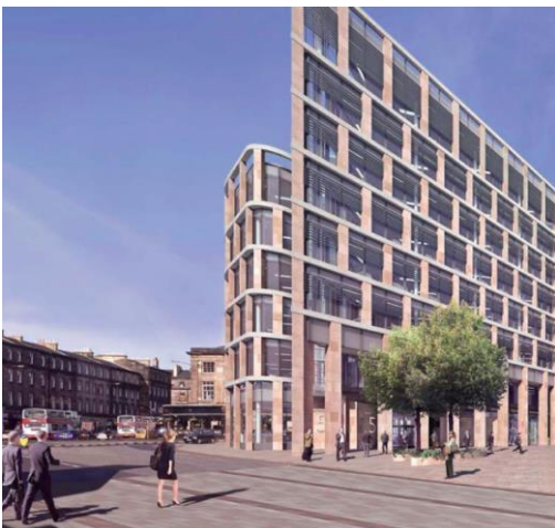
Construction fee – circa £200million Client: Interserve / Tiger Developments
