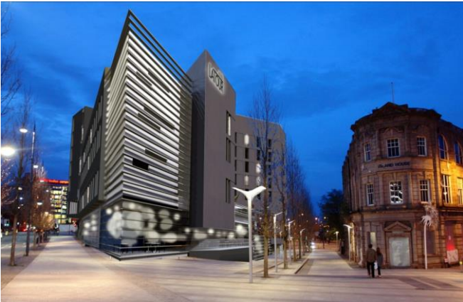
Construction fee – circa £20million Client: Hotel LaTour / Galliford Try
