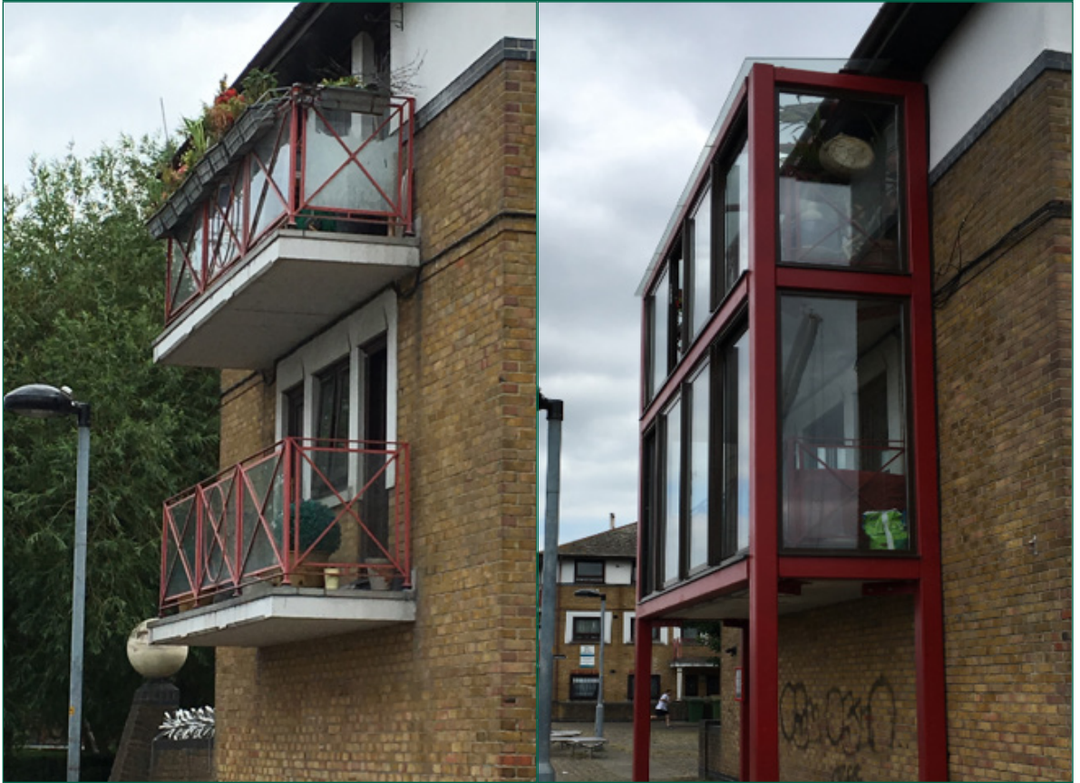
Figure 10: Balcony mitigation (before and after)
