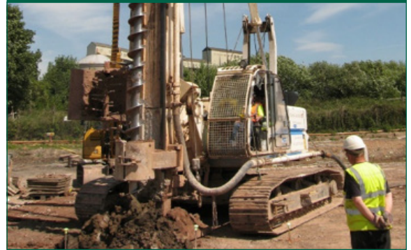
Figure 7: Use of Continuous Flight Auger piling produces less noise than other percussively driven methods
