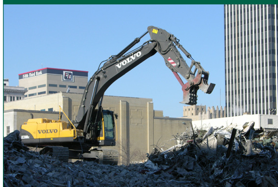
Figure 5: Use of hydraulic concrete shears instead of percussive breaking methods
