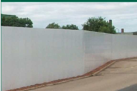
Figure 2: Purpose built site hoarding or perimeter noise barrier
