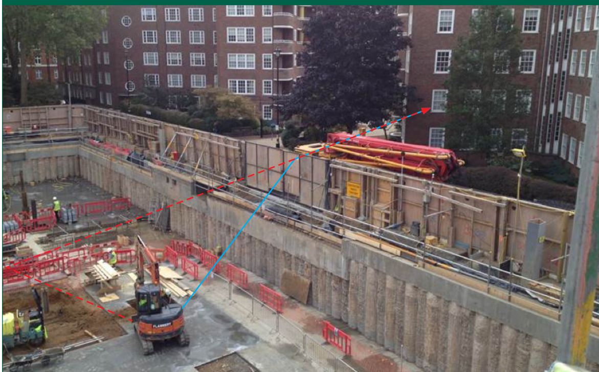
Figure 9: Example where the receptor does not have direct line of sight machinery but may be affected by reflections other structures
