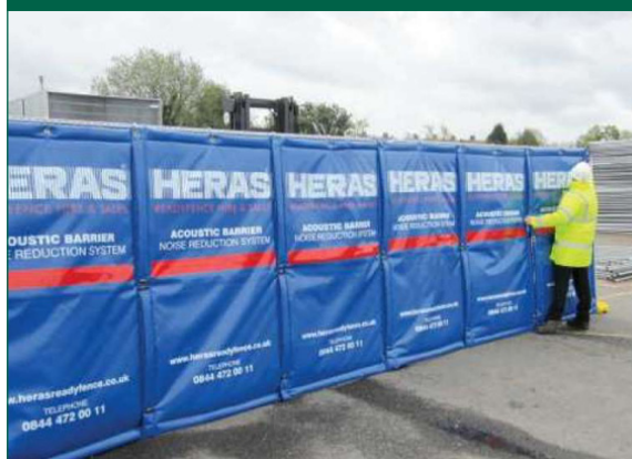
Figure 3: Localised temporary acoustic screening
