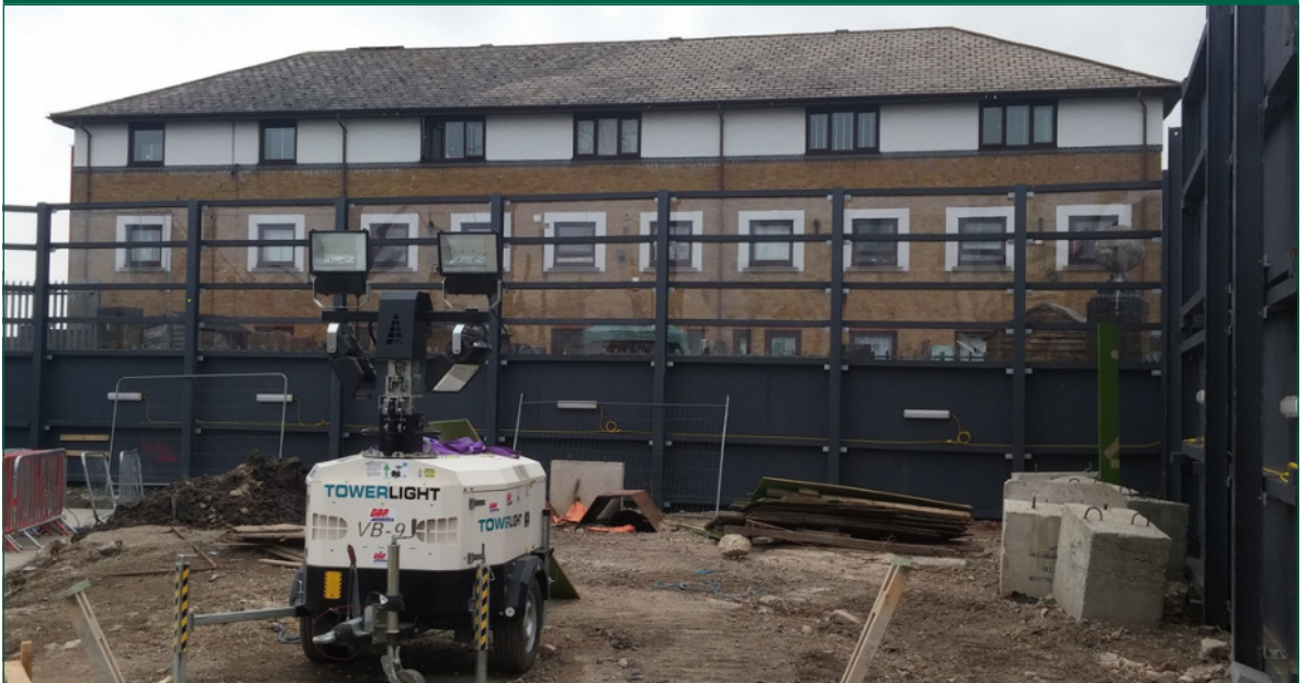
Figure 11: Construction hoarding incorporating a transparent upper section
